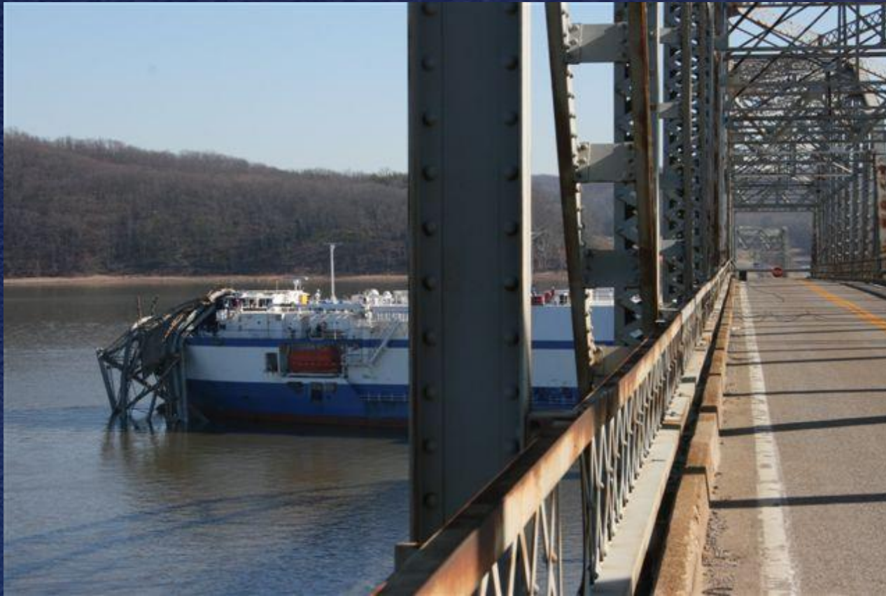
Cargo ship collision with highway bridge Marshall, KY January 26, 2012
